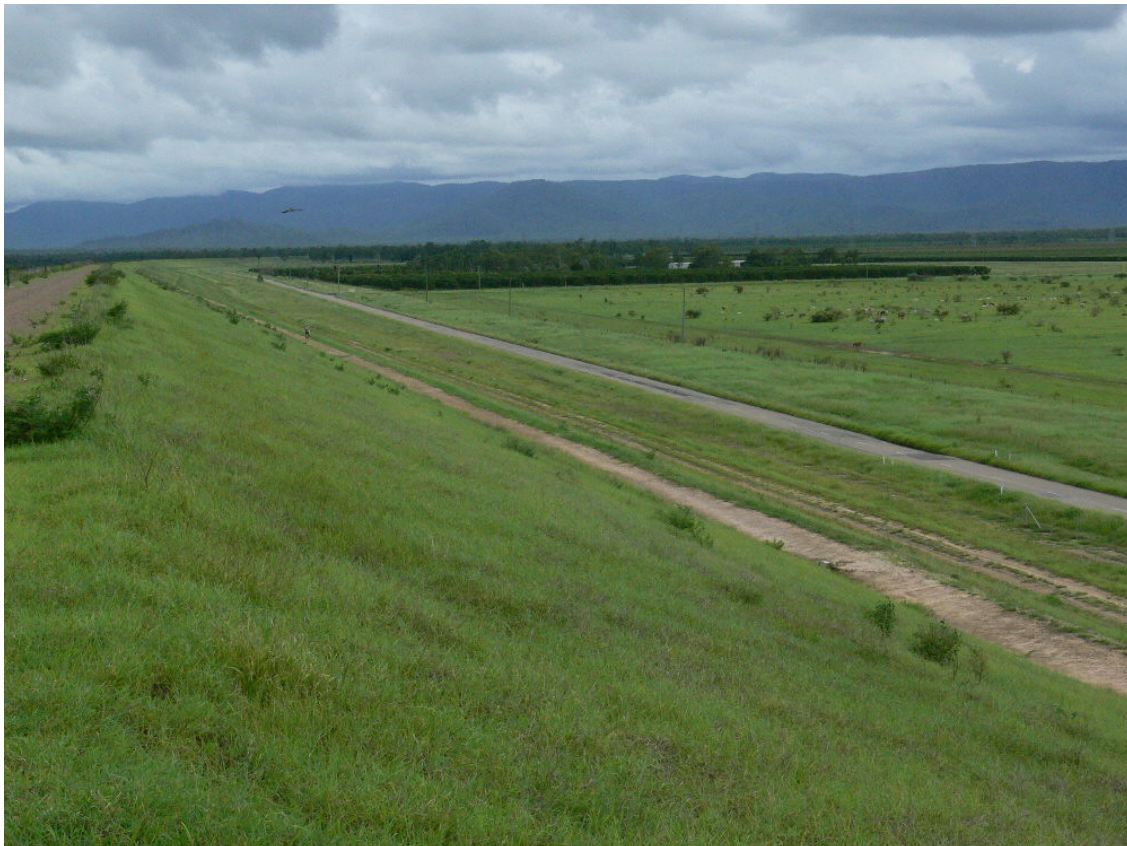
Figure 3.1 Ross River Dam Western Wall
