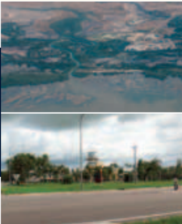
Top: Cleveland Bay Wastewater Treatment Plant is situated in a coastal wetland near Sandfly Creek.
