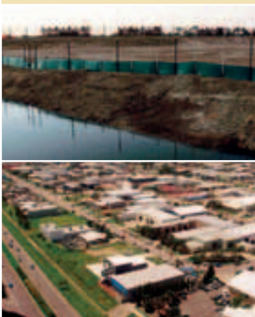
Top: Erosion and sediment control is necessary for all development and construction works.
