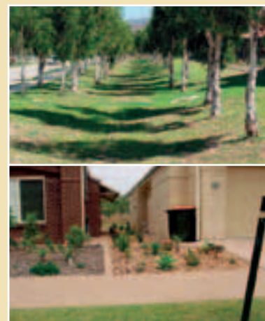
Top: Vegetated swale drains are a water sensitive urban design alternative to concrete pipes.
