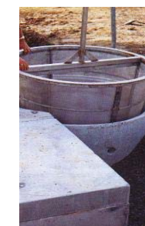
Many GPTs come in precast form, reducing construction times
