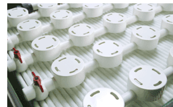
Figure 13a. Water distribution for a recirculating textile filter
