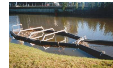
Floating traps are used in estuaries to capture highly buoyant material
