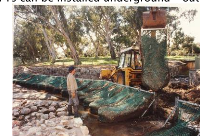
Nets can be used on open channels
