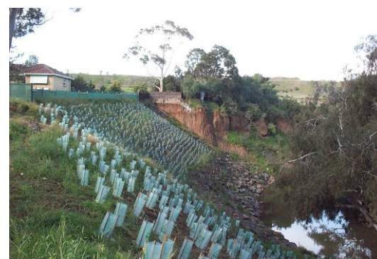
Riparian vegetation plays an important role in erosion control.
