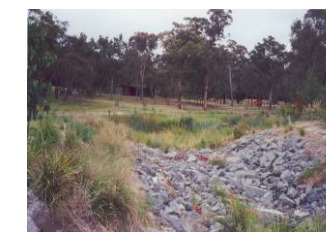
A high flow bypass is essential to protect vegetation
