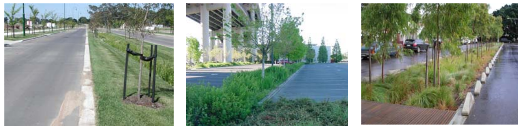
Buffer strip with flush curve without setdown
