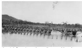
about 1.2 metres above the sand level. This successfully retained water which otherwise would have percolated down to the salt water section
